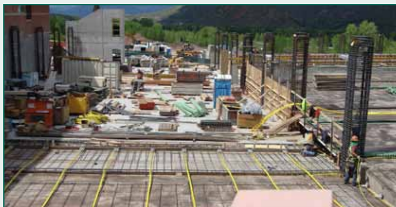
Preparing for the final concrete pour on the garage.
