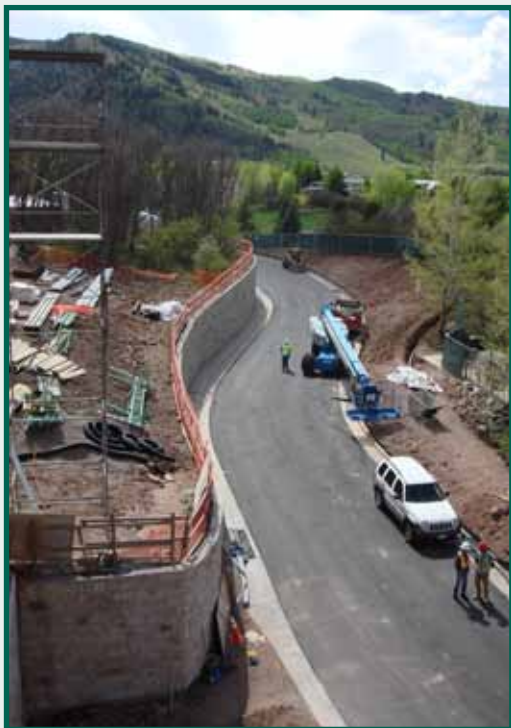
The "loop" road approaches completion.
